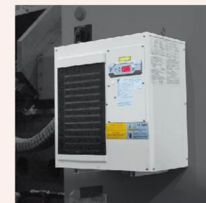
A/C for electrical cabinet
